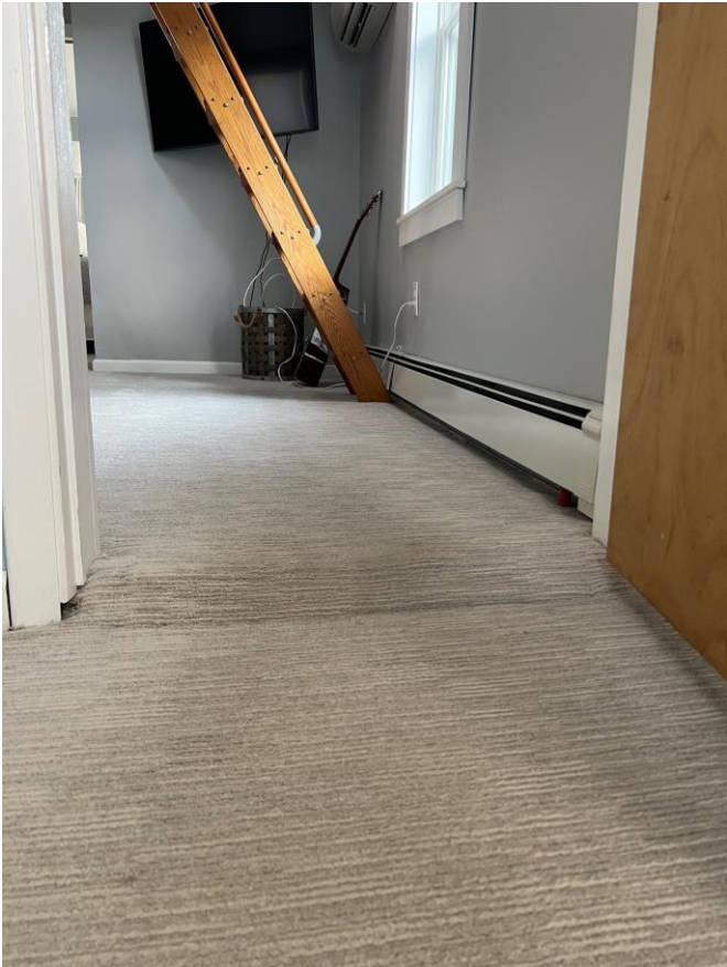
PHOTOS OF UNEVEN FLOORS ON THE THIRD LEVEL
